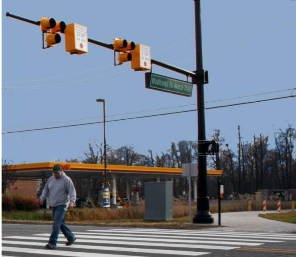
Fig. 9.71. Pedestrian Hybrid Beacon
