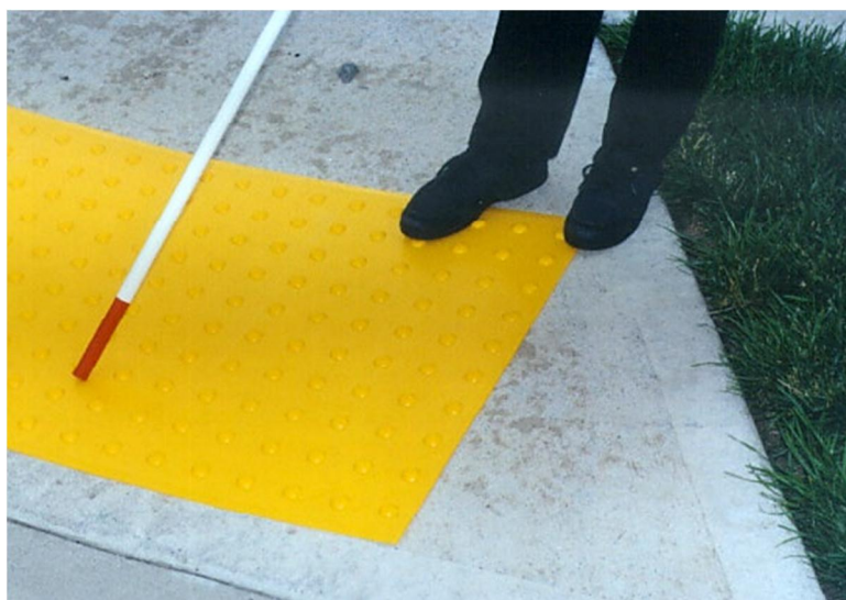
Tactile and contrasting color detectable warning strips provide pedestrians with vision impairments an important cue that they are leaving the sidewalk and entering a street.
