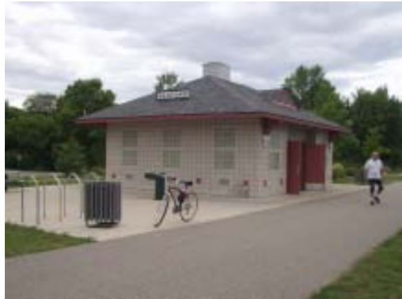
The Sanford staging area along the Pere Marquette Rail-Trail of Mid-Michigan has a depot themed restroom with numerous support elements. It also includes a community garden and historical interpretive signage.
