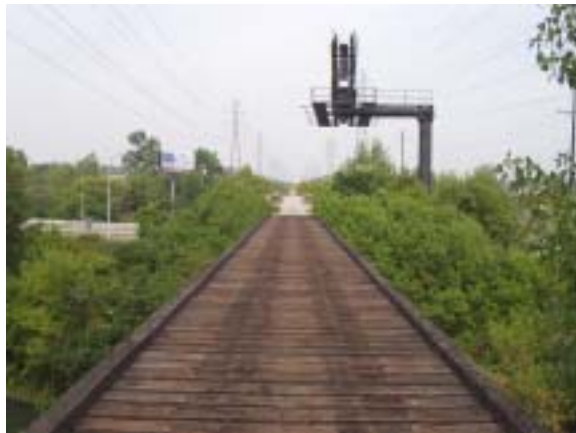
Northern Spur Rail Line bridge over the Clinton River
