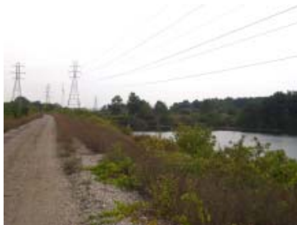
Looking south along the Northern Spur Rail Line just south of Auburn Avenue
