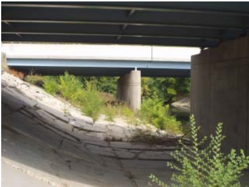
M-59 Bridge over the Clinton River looking north
