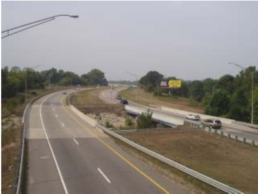
M-59 looking west from the railroad bridge
