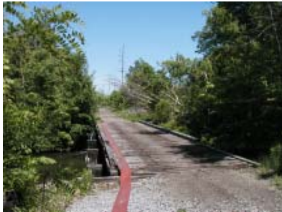
Existing open deck bridge over the Clinton River in Pontiac
