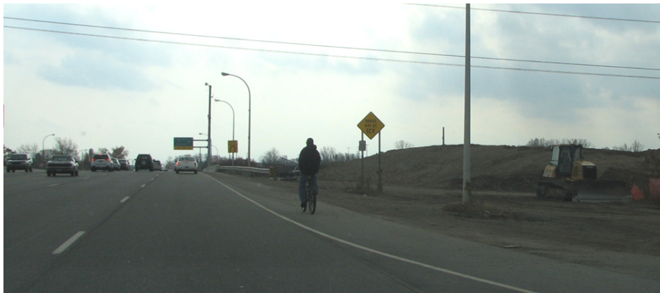
Existing conditions for the Novi Street overpass
