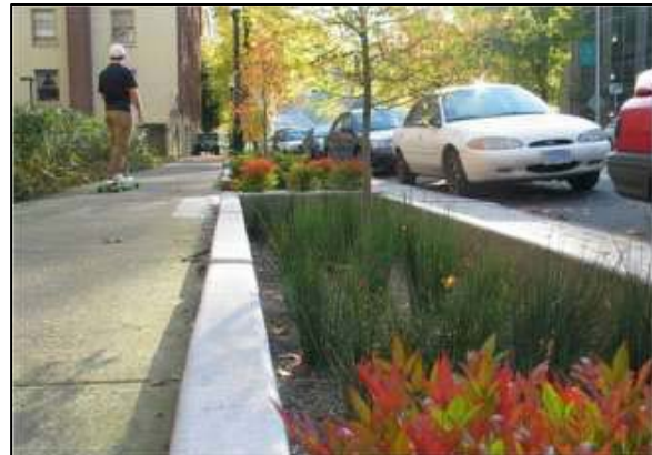
Example of using curb lawn to capture runoff while “greening” the corridor
