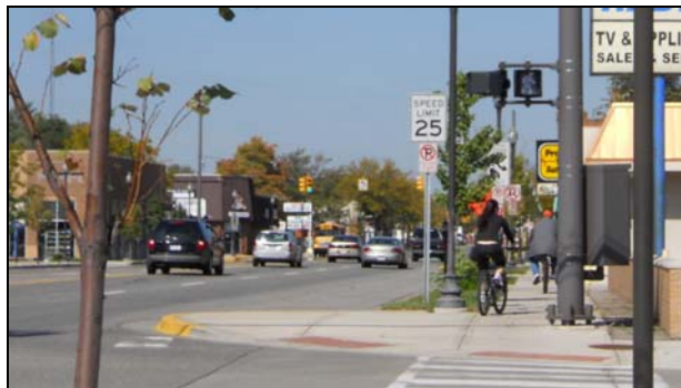
Although this street has sidewalks for pedestrians, there is no dedicated place for bicycles. A “complete street” accommodates all roadway users using context-sensitive design.
