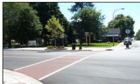
Example of how driveway design can draw attention to pedestrians in crosswalks.
