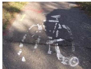
Painted markings require maintenance.
