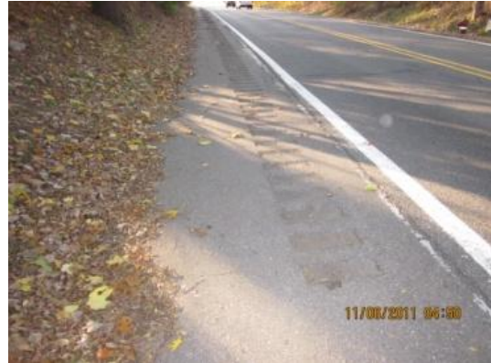
Despite this roadway shoulder's bike path designation, rumble strips to alert drivers of the road's edge were installed; interfering with pedestrian use.
