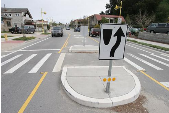
Raised islands provide a safe stopping point for pedestrians. Example: Santa Cruz, CA Source: Burden, 2011
