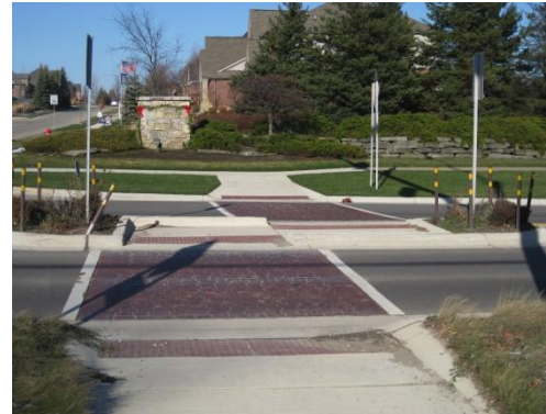
Decorative crosswalks and landscape can be incorporated into crossing islands. Example: Rochester Hills, MI
