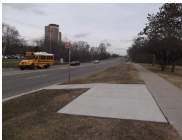
Additional concrete pads are being installed in City of Southfield.
