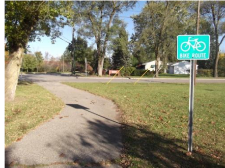
Class I: Independent riding surface separate from roadway
