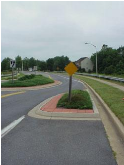
Roadway complete with landscape islands used as traffic calming measures. Source: Washington State Department of Transportation, 2012
