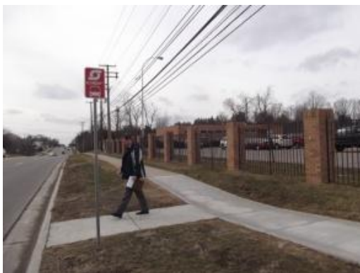
Properly installed keywalks enable safe bus access.
