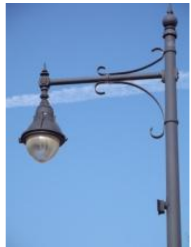
Downlighting can be used to illuminate sidewalks and bus stops. Example: Albion, MI
