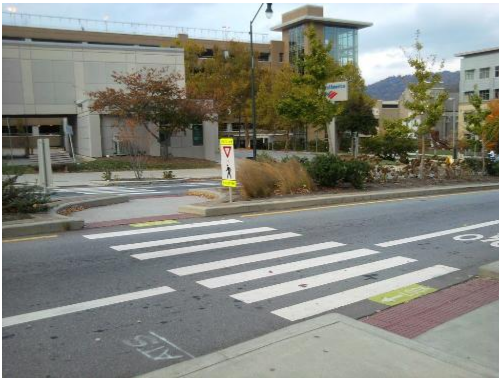
Adequate pedestrian crossing complete with cross markings, signage, and pedestrian harbor. Example: Asheville, North Carolina Source: Zuyeva, 2011
