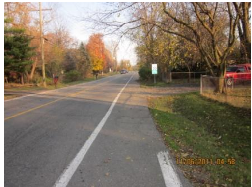
Paved Roadway Shoulders
