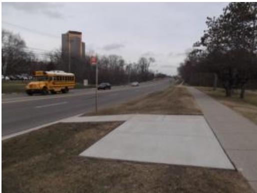
Newly installed concrete pad for future shelter.
