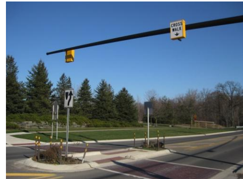
Illuminated crosswalk signs draw attention to crosswalk on a high-traffic roadway. Example: Rochester Hills, MI
