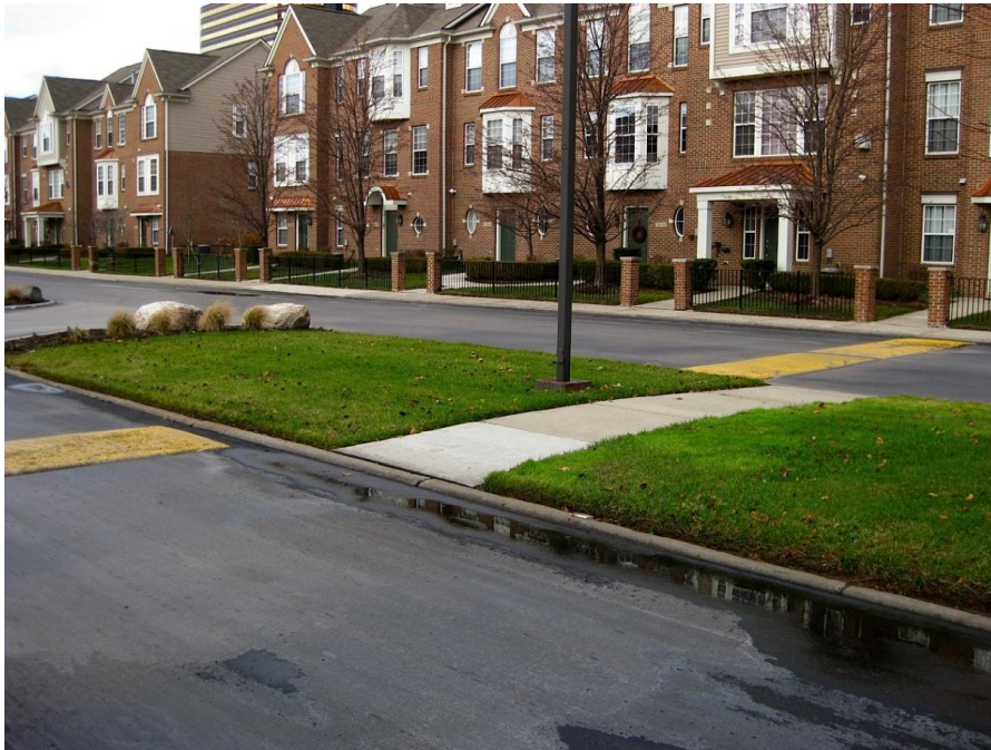
Roadway with speed bumps and median with pedestrian pathway in the Southfield City Centre District.
