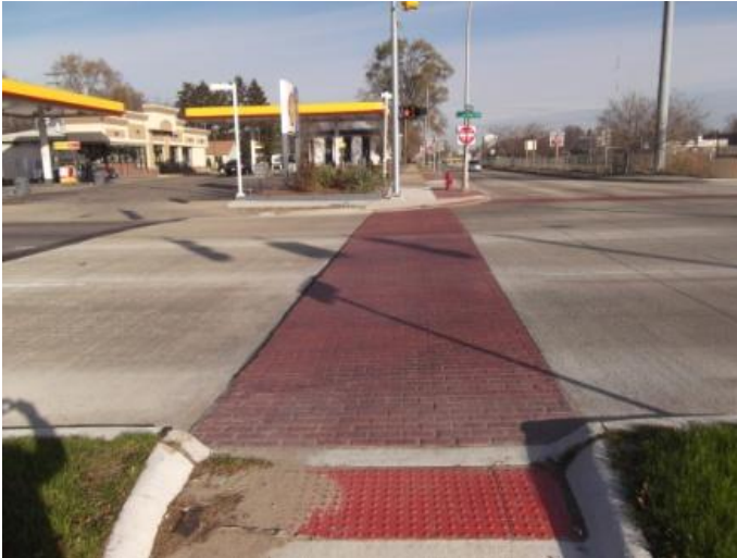
Defined pedestrian crosswalk with stamped concrete material. at 8 Mile Road and the Southfield Freeway.
