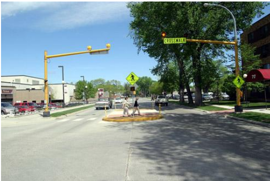
Overhead flashers help to define this crosswalk with raised pedestrian island. Example: Fargo, ND Source: Burden, 2011
