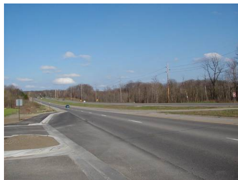
M-59 Corridor in White Lake Township
