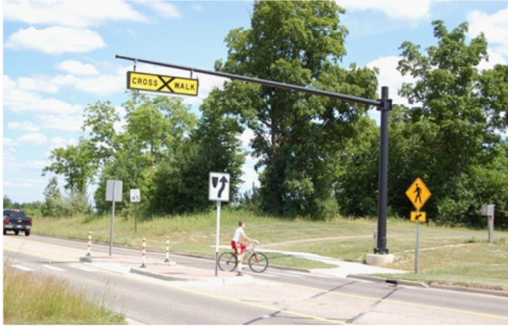
An overhead lighted crosswalk sign also provides illumination of a crosswalk on Oak Valley Drive in Scio Township, Michigan.
